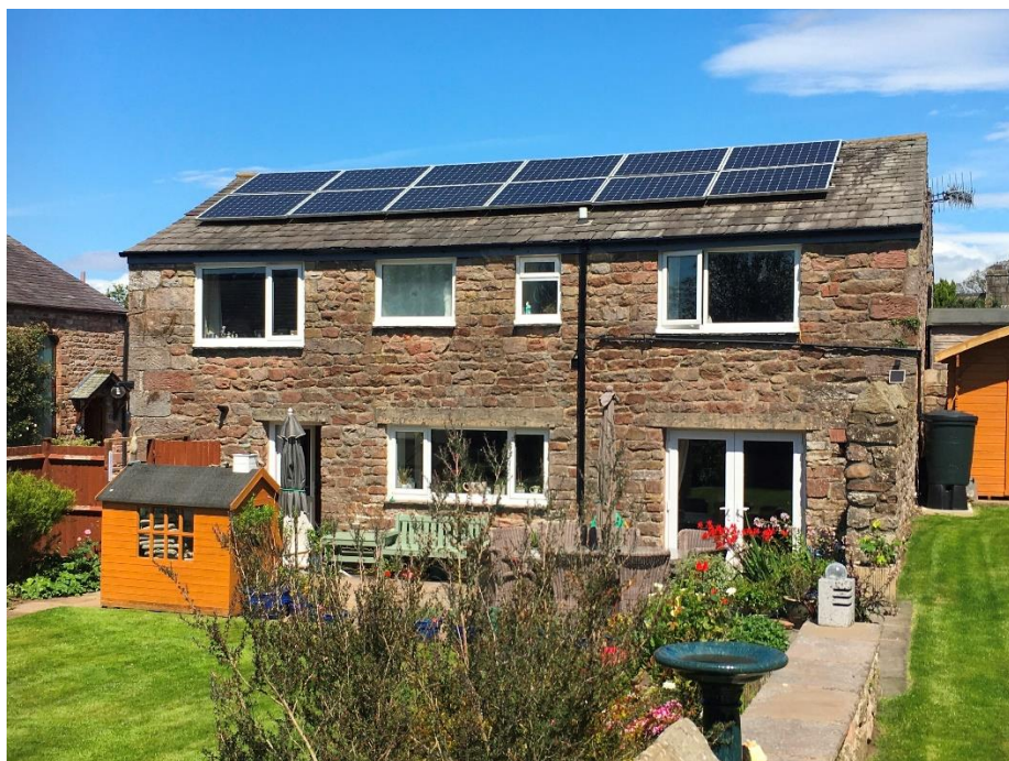
Solar panels on a house in Aldcliffe
